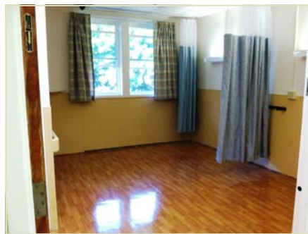
Patient room renovation
